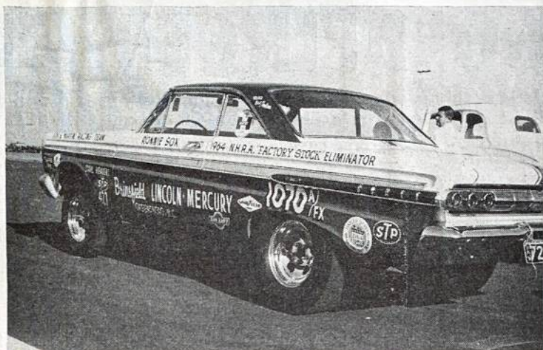
EXPERIMENTAL 7-litre Galaxie-engined Mercury Comet (above) covered the standing quarter-mile in the remarkable time of 11.78 secs.—better than most of the British racing cars! Sox had an exciting match-race with Dave Stickler's 7-litre Dodge. BOB KEITH works on his Chevylet-powered dragster, which did 9.54 secs. despite not coming up to expectations.
