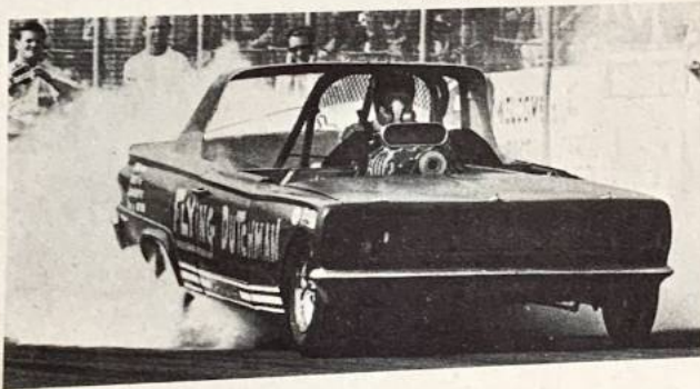
Below: Flame suit and mask to combat nitro fumes—the car is typical of the Funny Car class. It has a blown 426 Chrysler engine.
